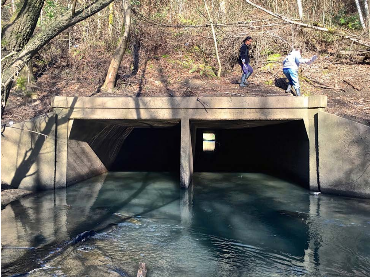
Figure 2.8 Culvert at Western end of property. Photograph by Rachael Gernhart 2016.
